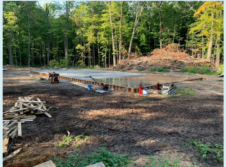
As approved by the electors: Slab poured for a new municipal storage building on Chambers Island
