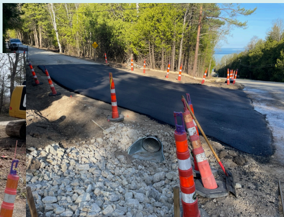
Above: New culvert placed on Islandview directing the water under the road instead of over it
