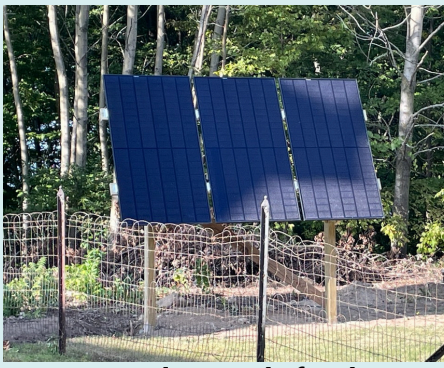
New solar panels for the lighthouse allowing 100 amp service. Previous service was just 12 volts!
