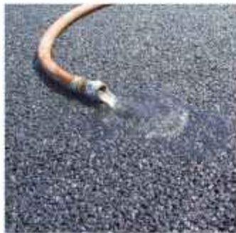
Figure 40. Paving bricks or a mix of asphalt or concrete with pores for water to soak through and reduce storm water runoff
