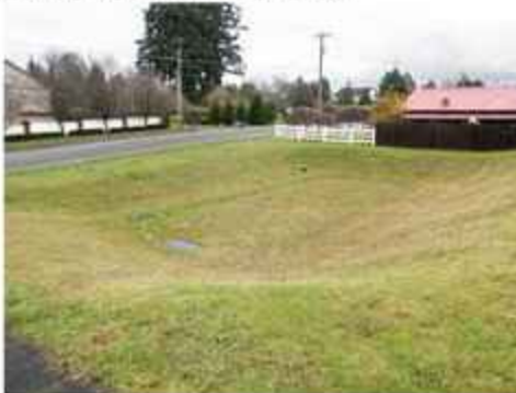
Figure 41. Small grass stormwater basin infiltrates runoff
