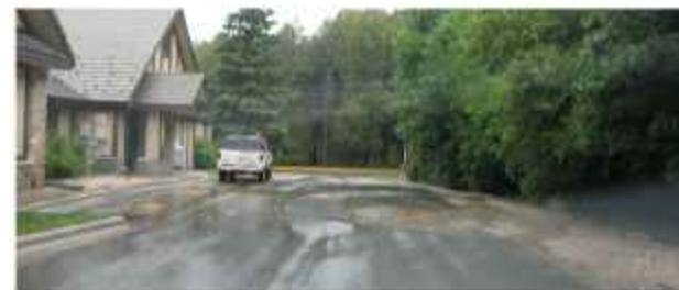
Figure 27. Stormwater runoff is a concern at the Town Center.
