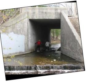
and restoring the creek bed, as well as, the development of an above-grade walkway adjacent to the creek, designed to allow for safe passage below Highway 42 during low flow by people and wildlife.
