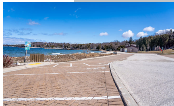
Porous pavement and natural berm in the Village of Egg Harbor to prevent runoff and decrease water contamination, Rachel Lukas, Door County Pulse
