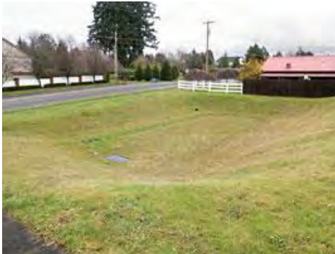
Figure 41. Small grass stormwater basin infiltrates runoff
