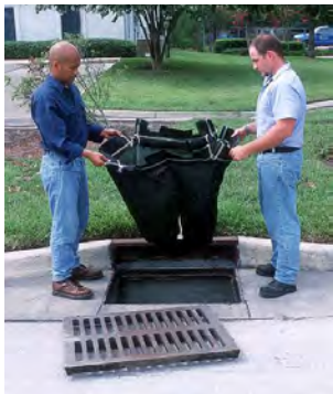
Figure 39. Catch basin inserts trap trash, sand, silt in runoff before entering pipe system
