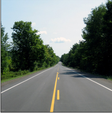
Portions of County Highway A provide paved shoulders that are adequate for bicycle use.
