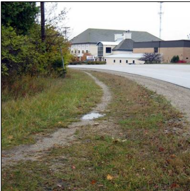
"Desire lines" across from Gibraltar School indicate heavy pedestrian usage and a need for sidewalks.
