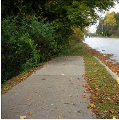
Sidewalks abruptly end along Highway 42 in Fish Creek without extending approximately 1/3 mile to Gibraltar School.
