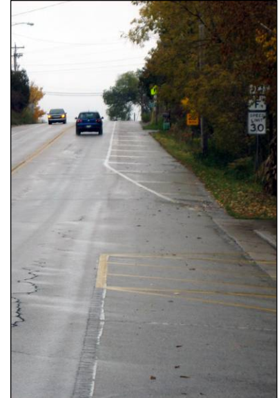
Adequate space exists for bike lanes on Highway 42 traveling from downtown to Gibraltar School and the YMCA.
