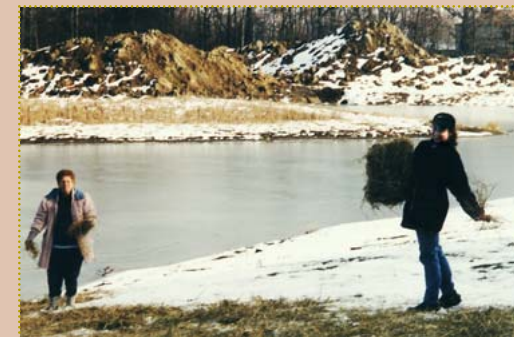
The site was hand mulched after seeding and planting.
