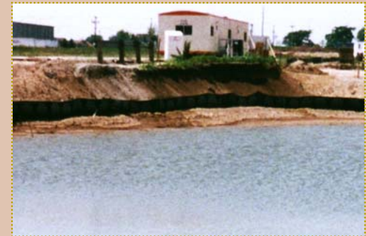
Construction site in summer of 1999.
