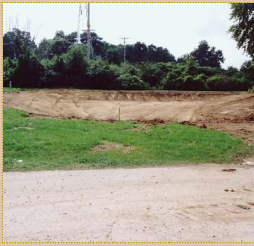
Infiltration trench during construction and seeding.
