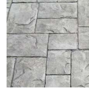
STAMPED CONCRETE : ASHLAR STONE
